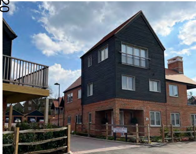
Example of a key building
