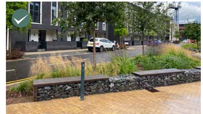
Use of gabion walling as a feature in the public realm - could be used to create elements of protection and enclosure as well as seating.
