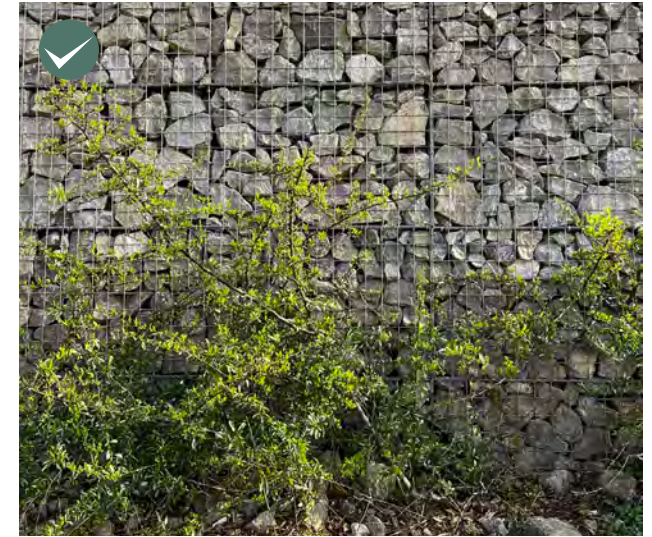
High-quality gabion retaining wall with additional planting
