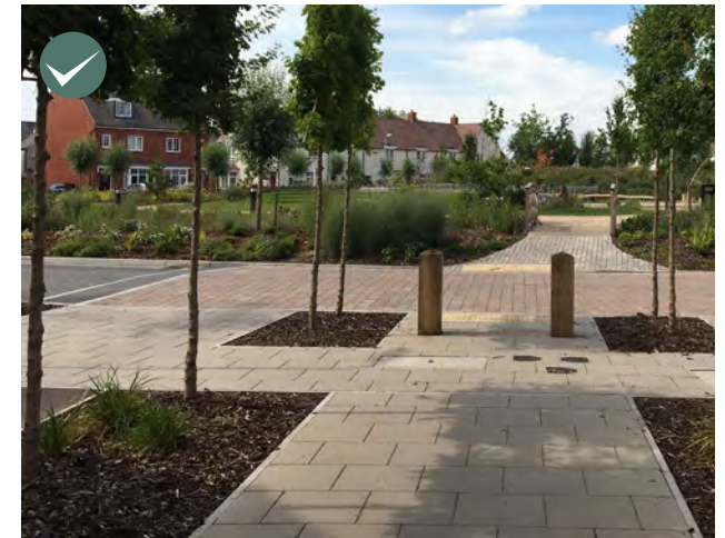
Junction between a street and a footpath where a raised table and textured paving gives clear priority to pedestrians
