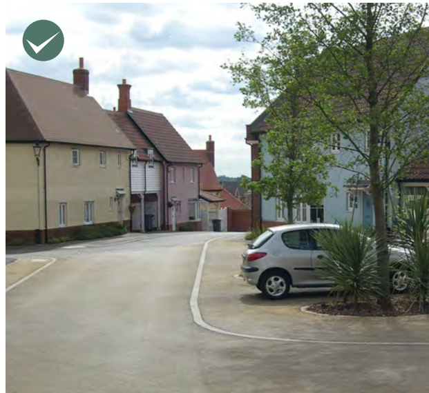
Tight junction radius and raised table
