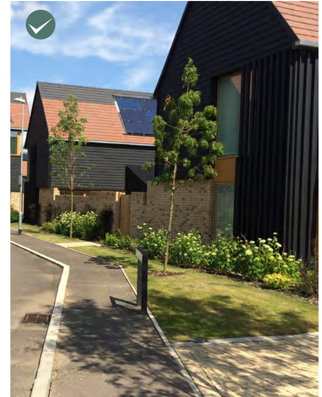
Dwellings with side gardens, active frontage onto the street and no rear windows with a planted boundary complementing the built form.
