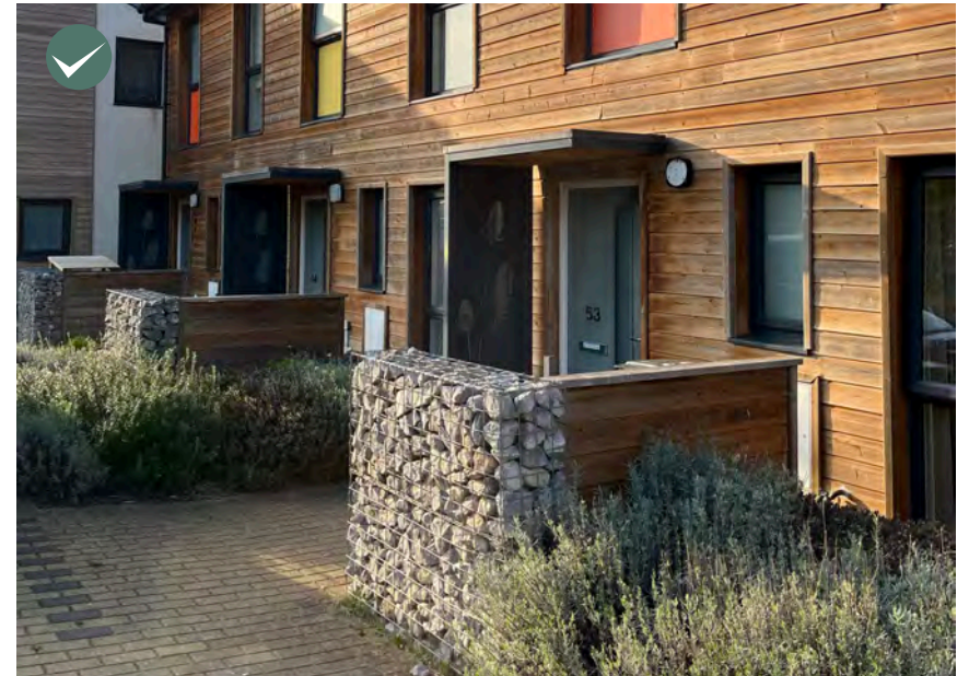
Use of natural materials and front boundary gabion walls that matches retaining walls across the site
