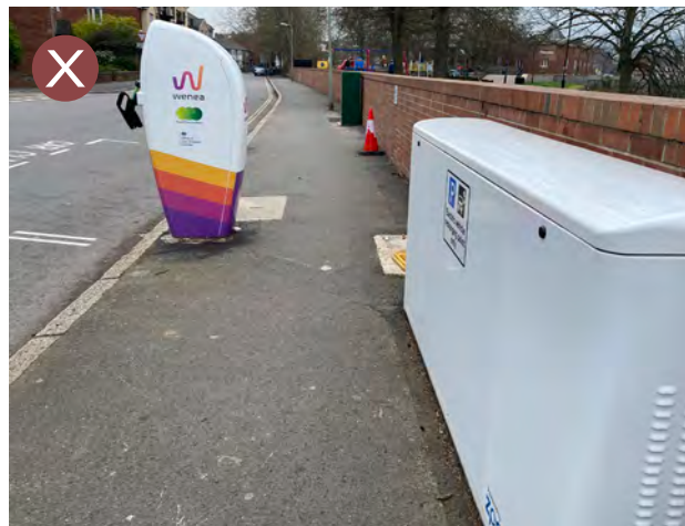
EV charging point obstructing footway and with visually intrusive design and size
