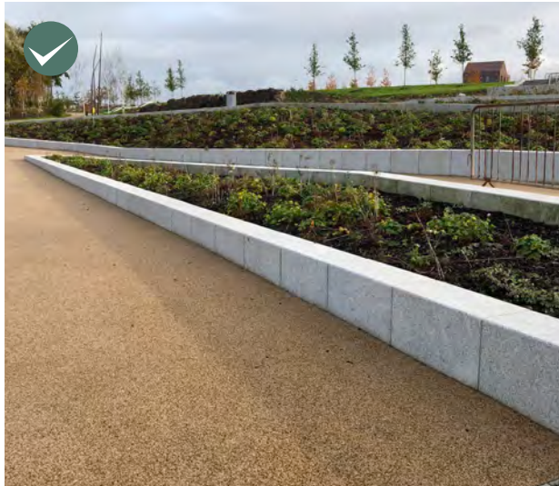
Use of landscape features to deal with level changes - opportunity to be innovative.
