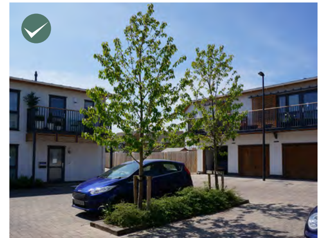
1.5m wide verge with rectangular shaped planting area to allow sufficient space for trees
