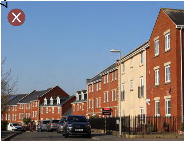
Inconsistent roof line and massing
