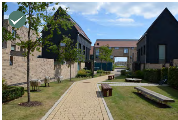
A focal point with marker building and play features defining the threshold between the space and the development
